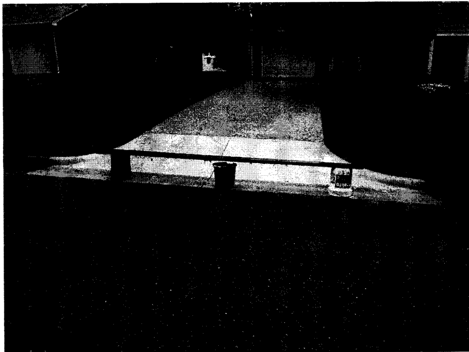
Figure 2 - After construction of standard concrete driveway entrance gutter
